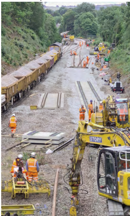
Laying new track
