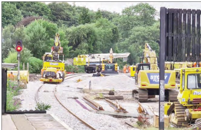
Laying new tract at Dore & Totley Station
