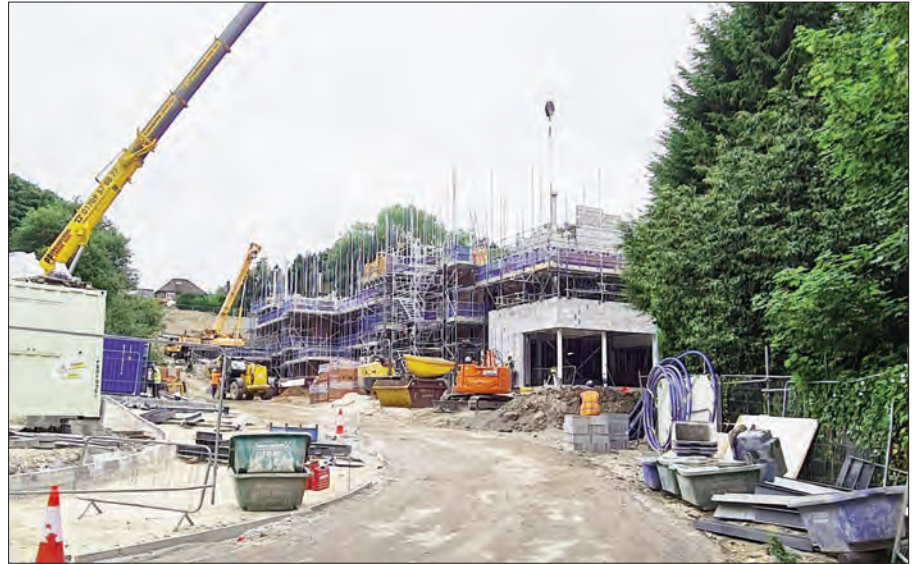
Work on Outram Fields reaches the third storey.
