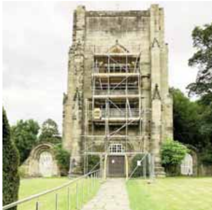
Scaffolding on the Abbey Tower
