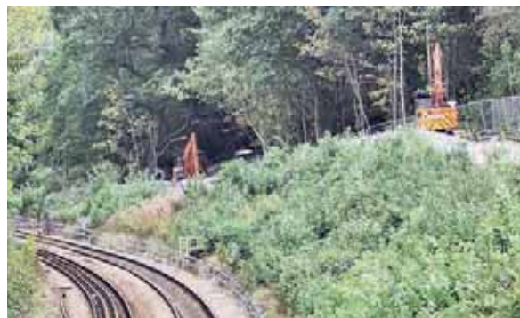
Work starting on the Poynton Wood site
