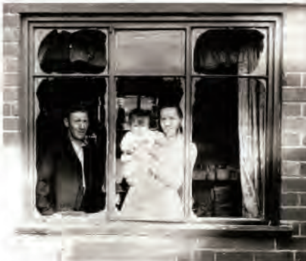
Shattered windows. Surveying the damage
